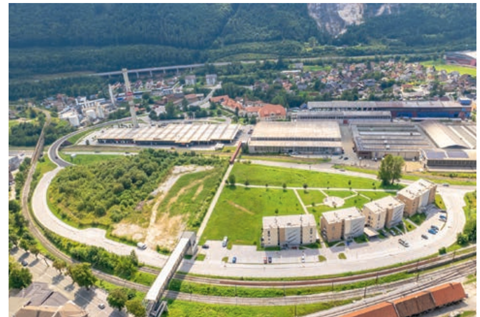
Hrenovca area today, 2023 (photo by: Gregor Vidmar)
