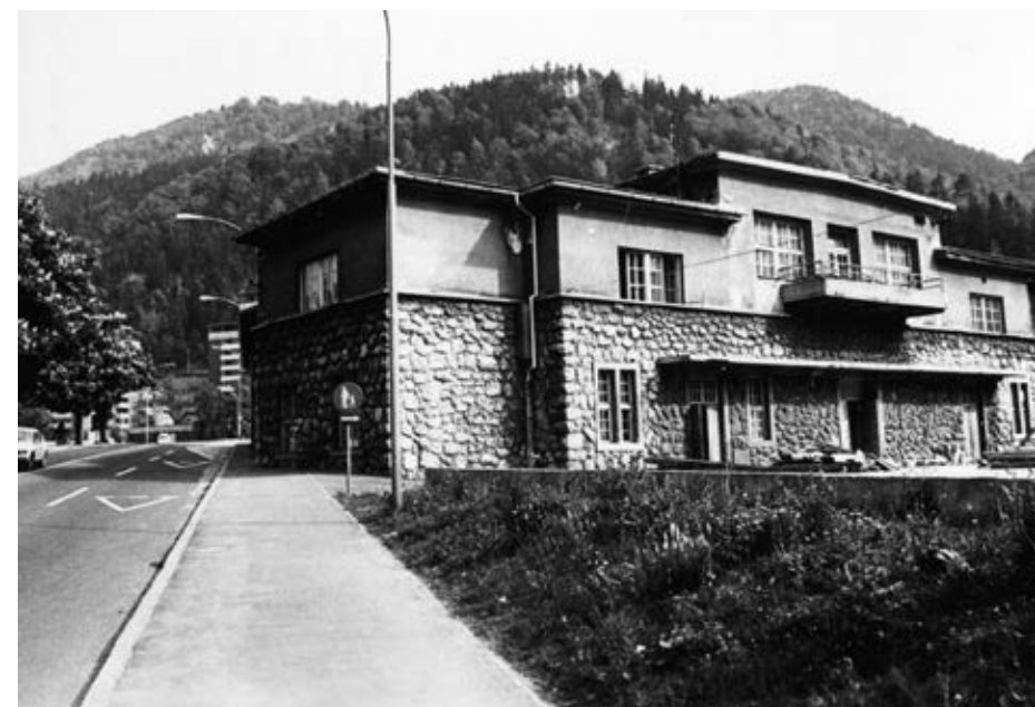
TVD Partizan (Physical Education Society Partizan). Jesenice building from the south, 1979 (archived in the Photographic library of the Jesenice Upper Sava Museum)
