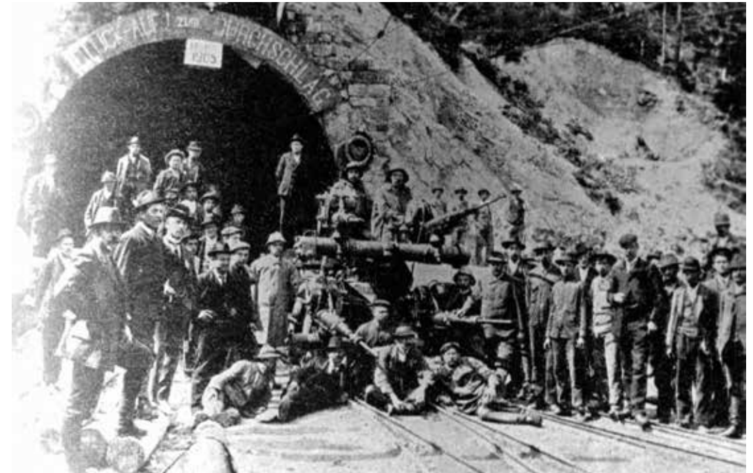
Workers celebrate the breaking through of the Karavanke tunnel on the Karavanke–Bohinj railway in 1905.
